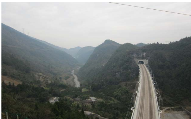
The Yichang-Wanzhou railway crossing Sanli township
